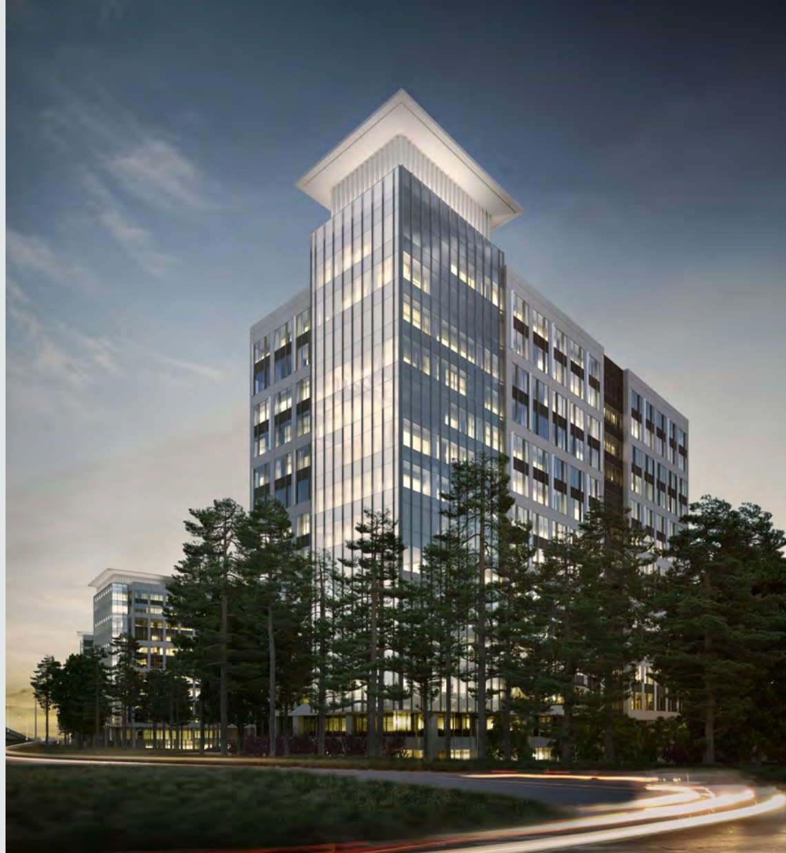
View of Phase I from Hardy Tollway
