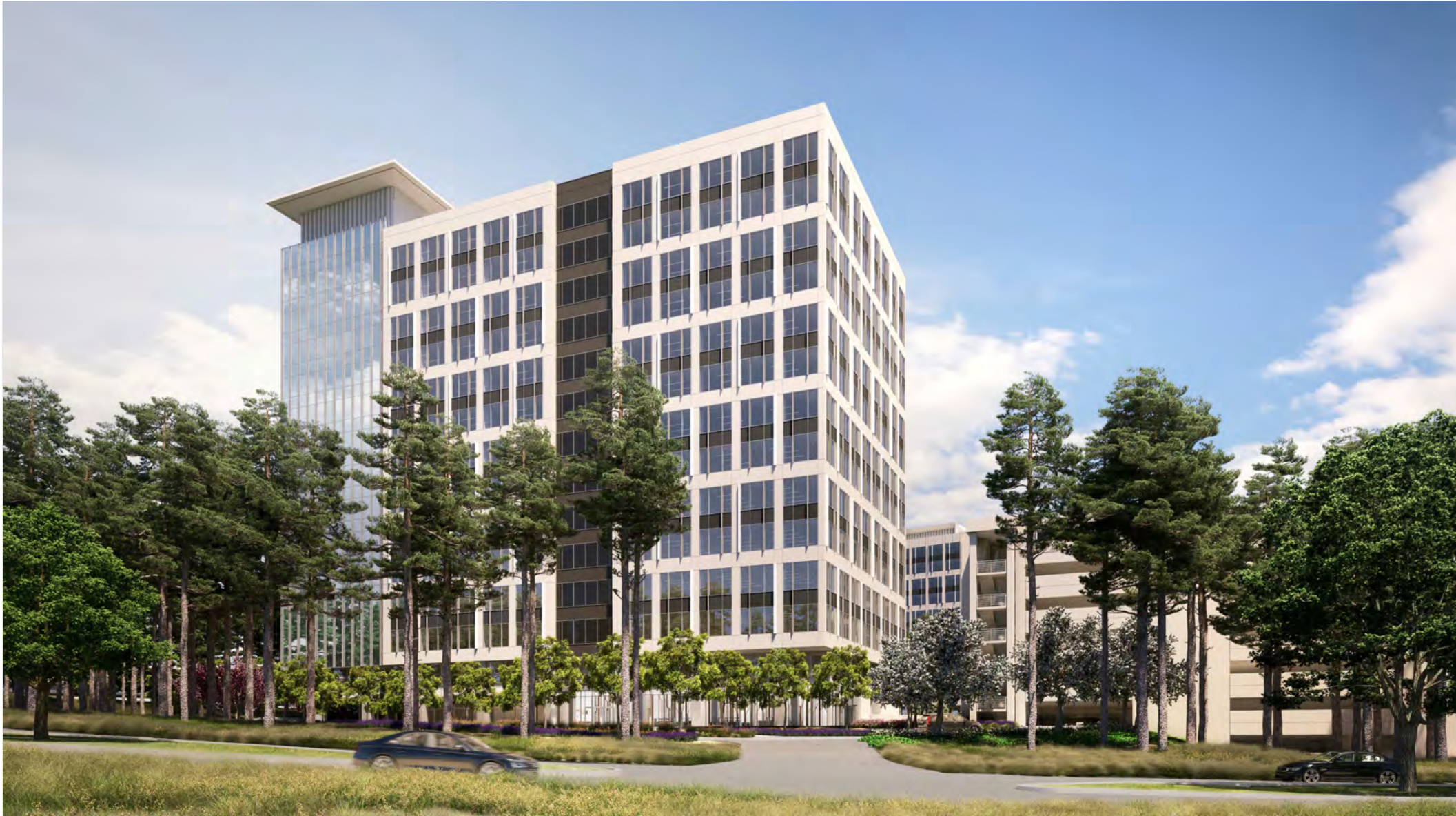
View of Phase I from Springwoods Village Parkway
